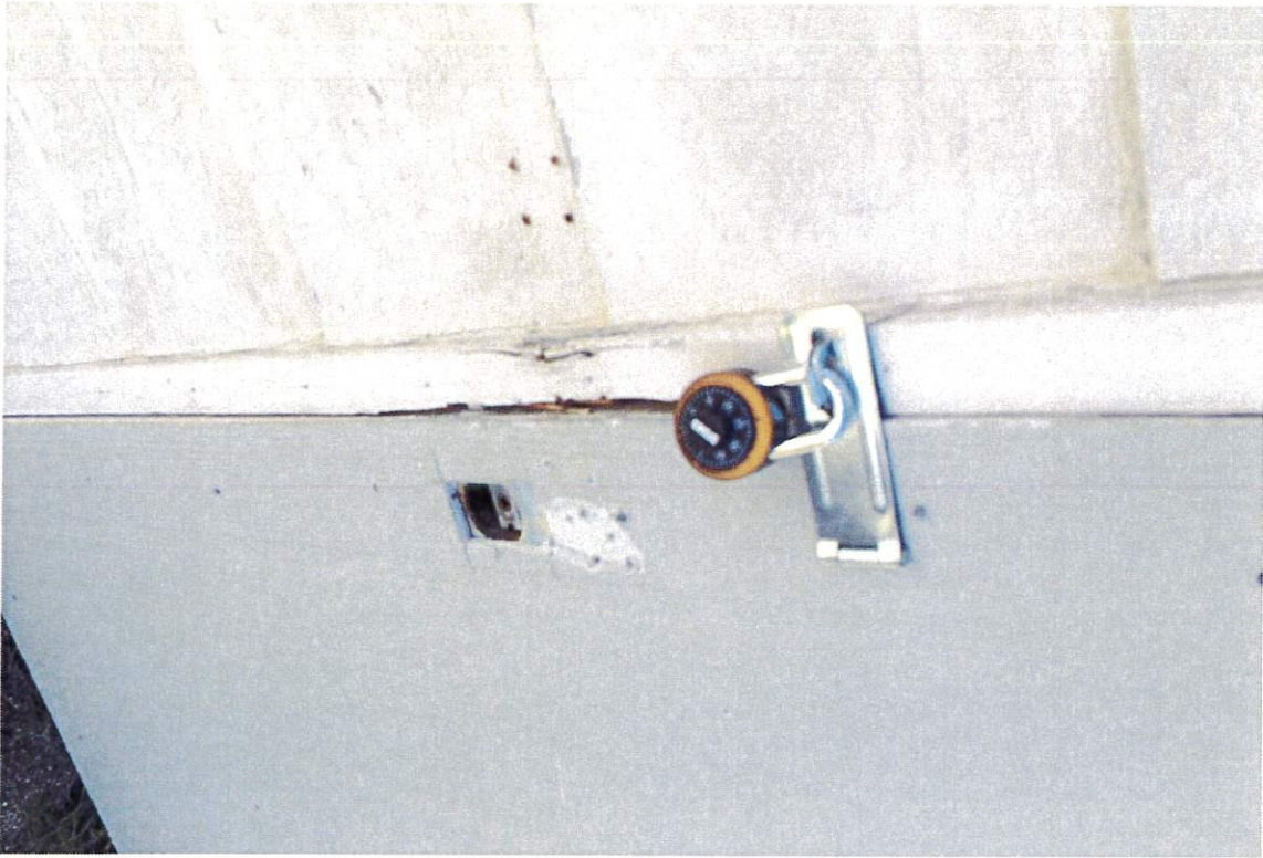
Well #2 New Lock
